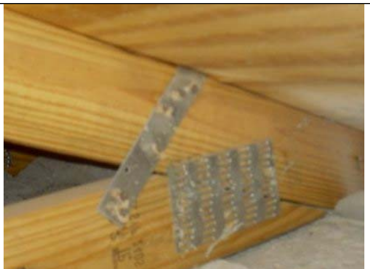
Roof to wall attachment
