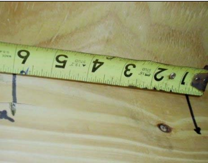
Roof deck attachment
