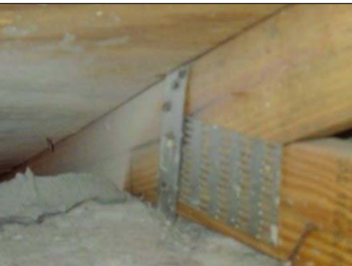
Roof to wall attachment
