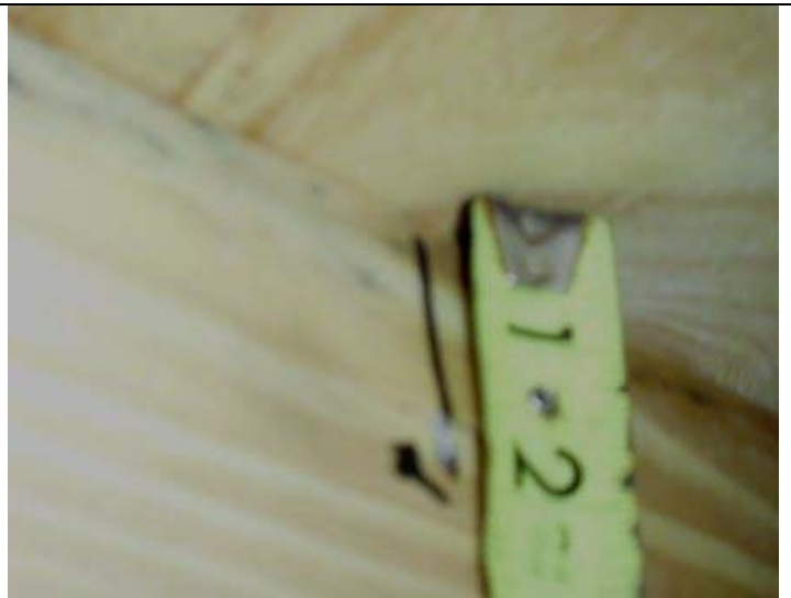
Roof deck attachment
